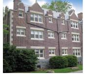
Repointing of the brick and stone facade was required in many locations due to the deterioration of the existing mortar
